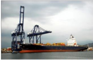
2 Quayside Post-Panamax Gantry Cranes
