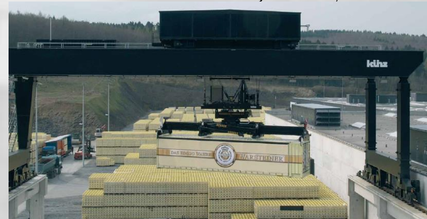
Automated RGC at Warsteiner, Germany
