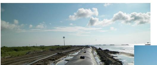
5,300 Linear Feet 30' diameter geotube 10'completed dune height
