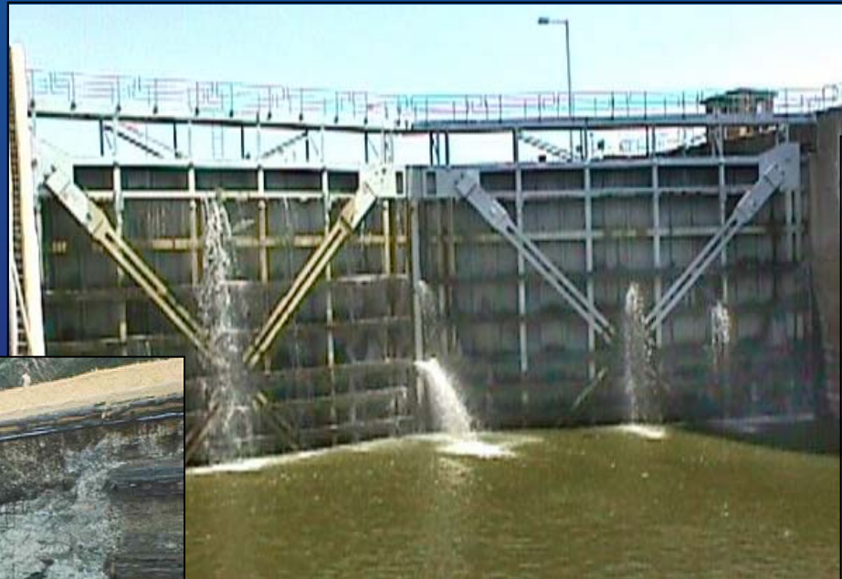
Leaking miter gates, Upper Miss Lock 19
