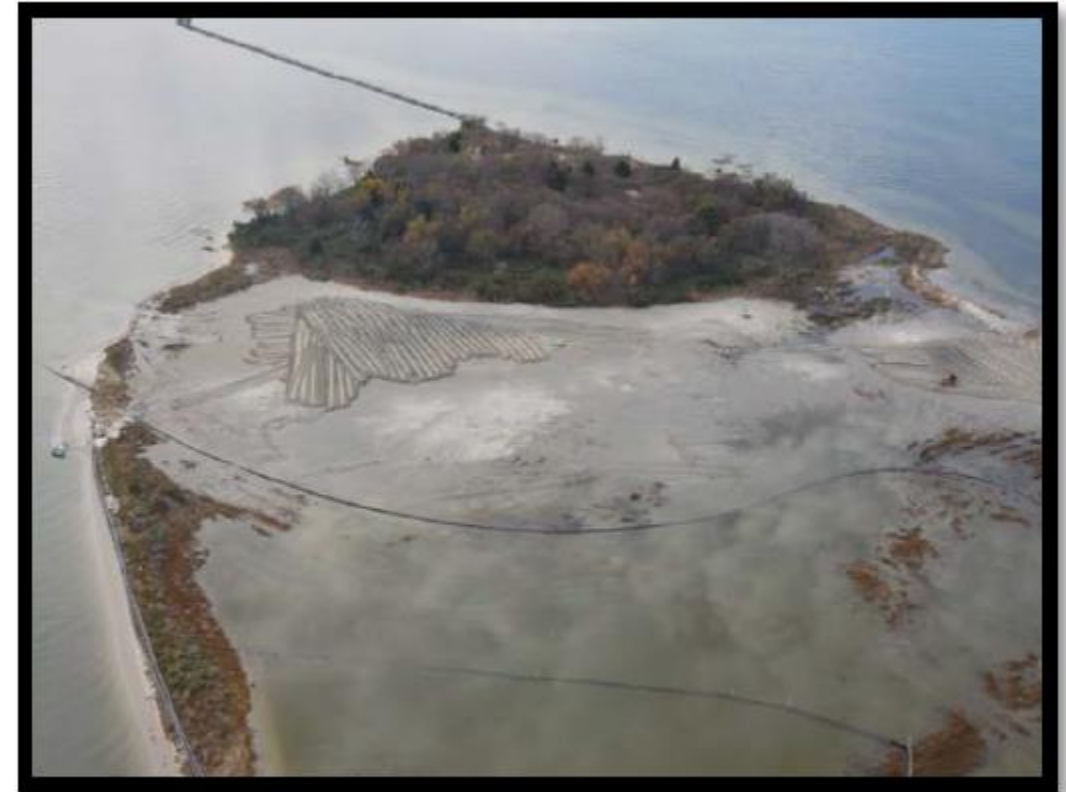
Dredging material (beneficial use), - Swan Island project
