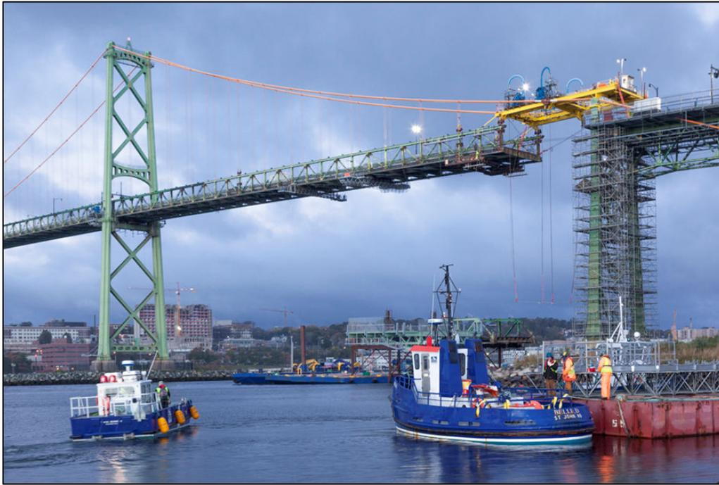
**Figure 1 – Deck Segment D1 Being Replaced**
