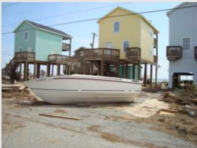
Hurricane Ike damage (Source: NOAA)
