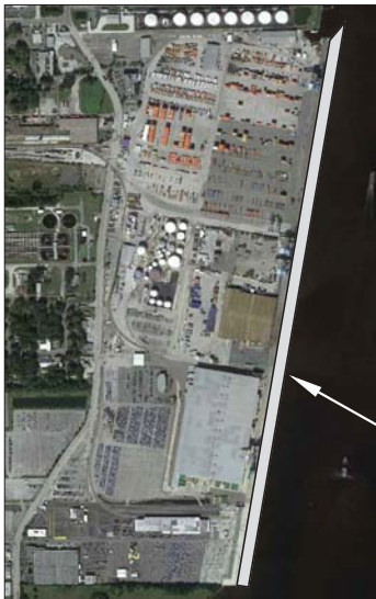
TALLEYRAND MARINE TERMINAL
